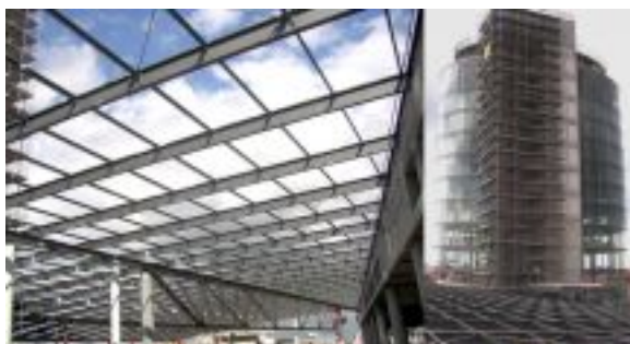
DaimlerChrysler AG, New Branch Munich, Delivery and assembly of completely welded construction View image
